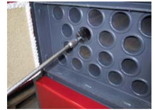
Cleaning the tubes
